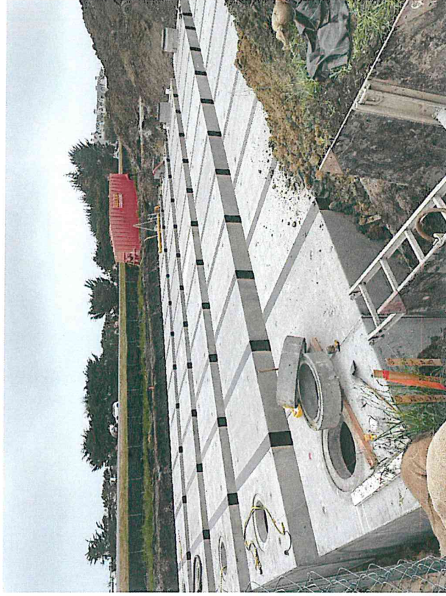
Chamber Assembly Completed
