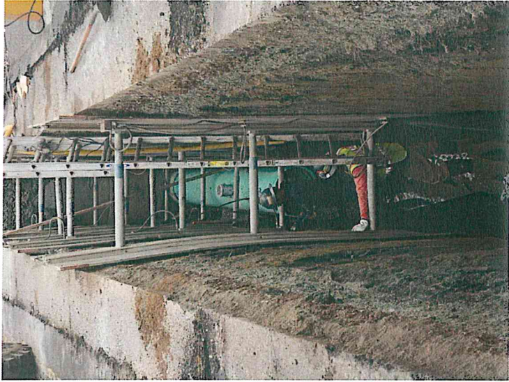
Installation of (N) 24" Sewer Pipe
