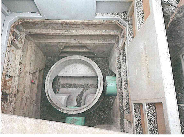
Installation of (N) Manhole
