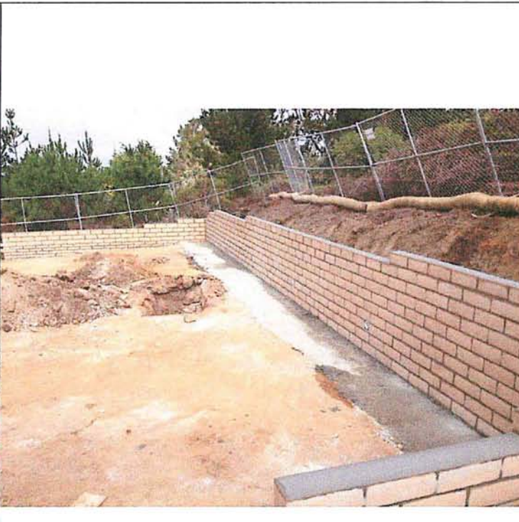
Masonry Retaining Wall Complete
