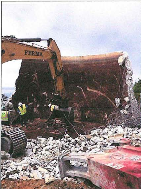
Demolition of Old Concrete Tank
