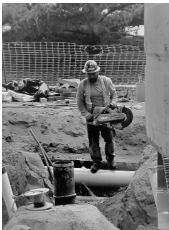
Installing a new water main at 16th Street & Cabrillo Highway. October 2018
