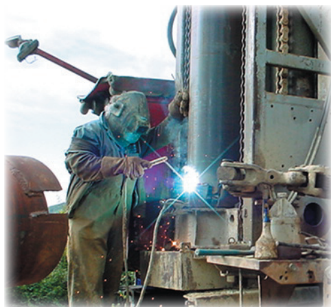
Installing a 12" steel casing in the new Alta Vista well
