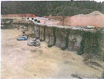
Begin shoring first "lift" downward
