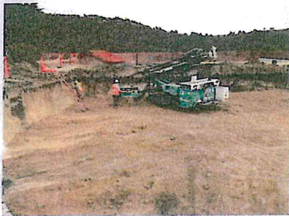
Shoring wall tie-back installation
