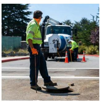
Sewer flushing truck in service
