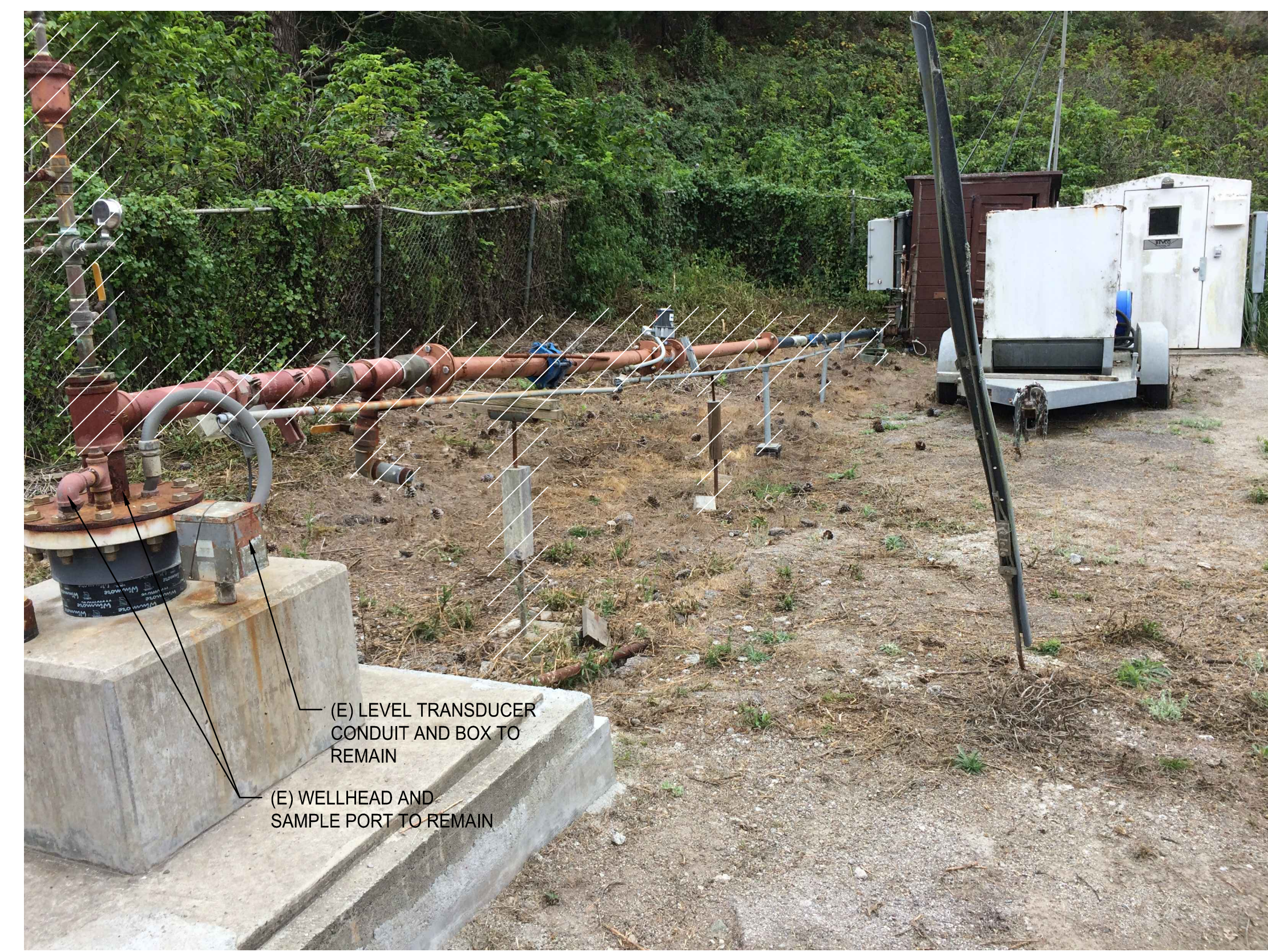
2 (E) WAGNER WELLHEAD DEMOLITION PHOTO Scale: N/A
