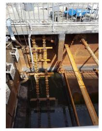
**Project:** 2.12 WWTP – Replace chain and flights and collector gear reducer in primary
